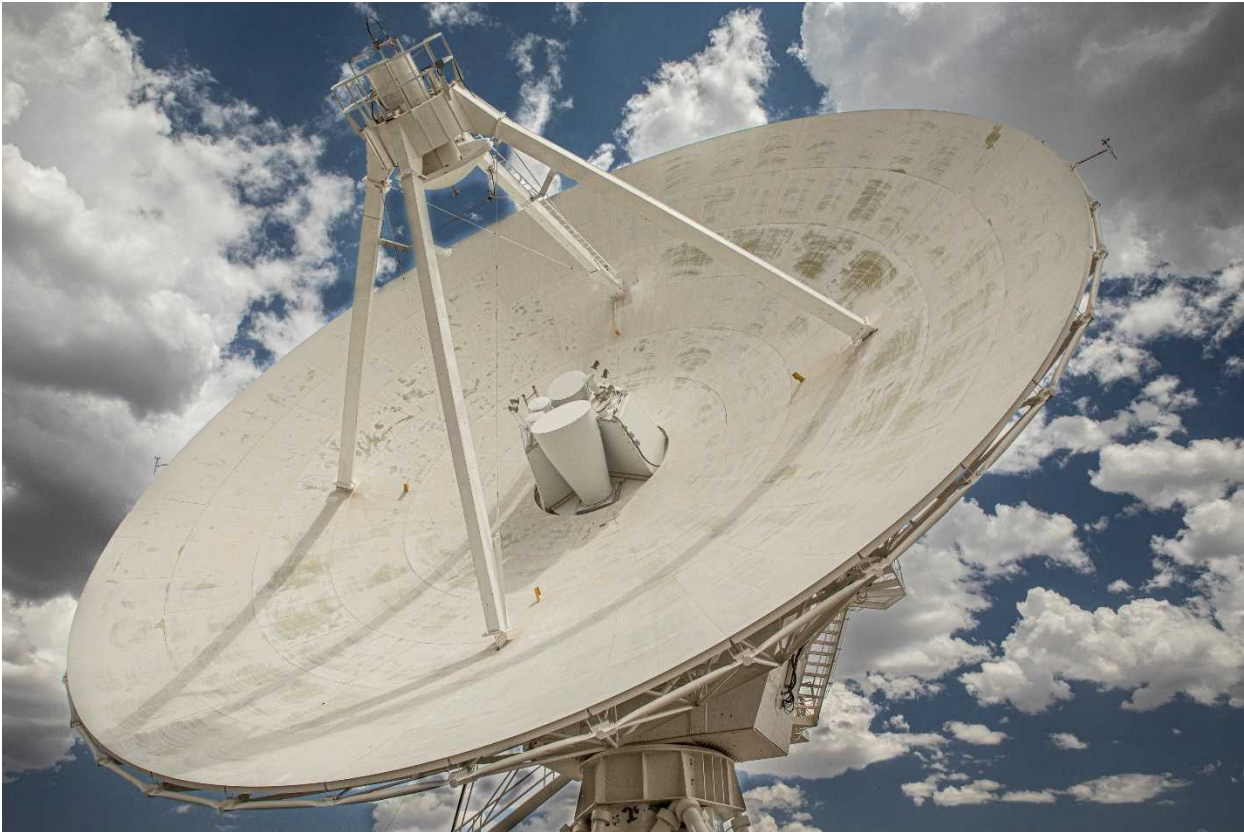
VLA Radio Telescope Dish – Receivers in Center (Photo from Visit)
